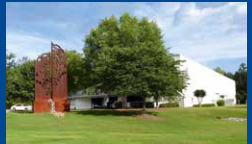
RAS Systems LLC in Georgia, USA
