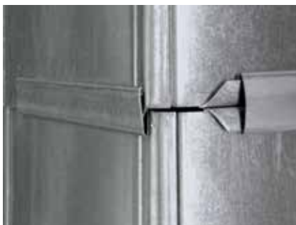
„S“ seam and drive cleat
