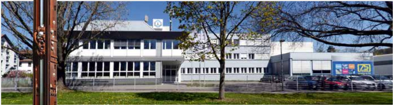
Headquarters in Sindelfingen. In the foreground „Steel object“.
